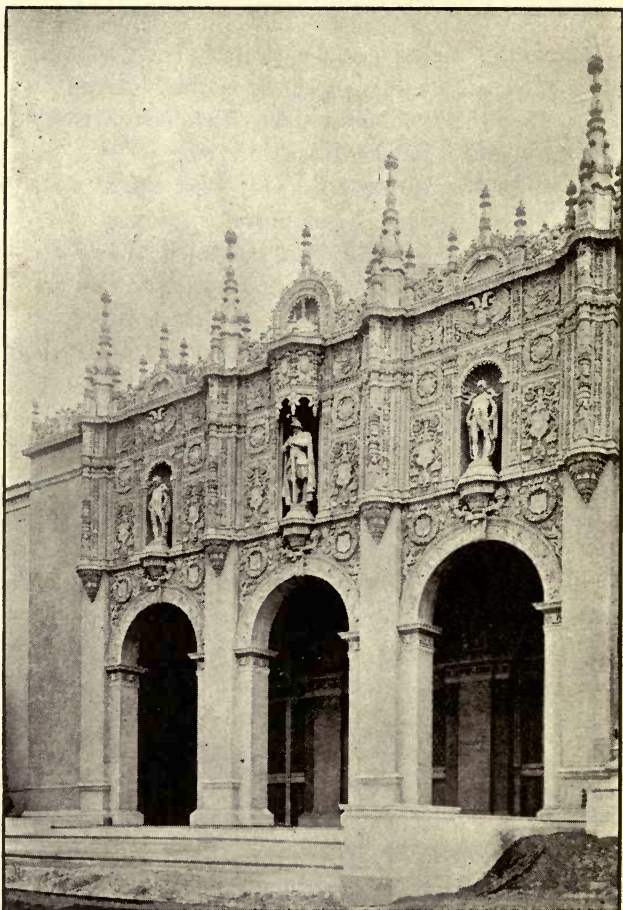
THE PORTAL OF ALL THE PALACES FACING NORTH By W. B. Faville
